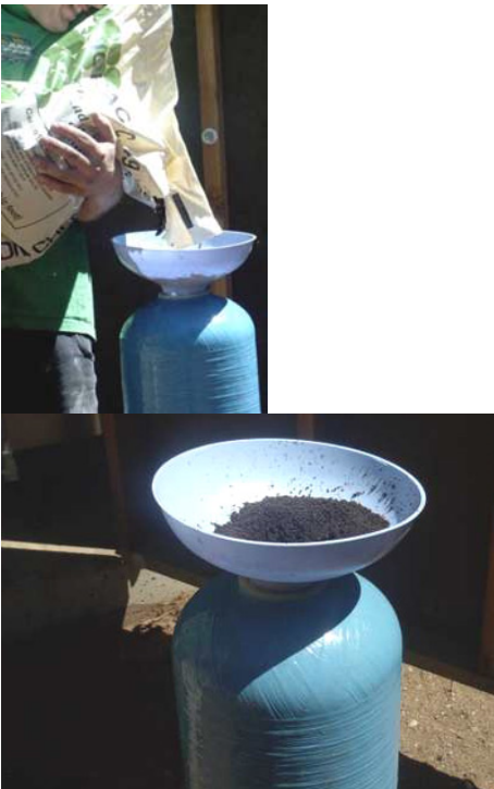
Adding media to the tank.
