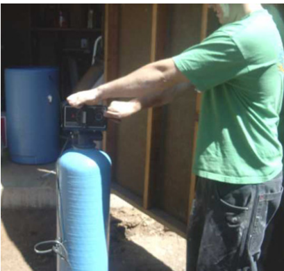
Screwing valve onto tank.
