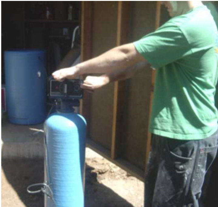
Screwing valve onto tank.
