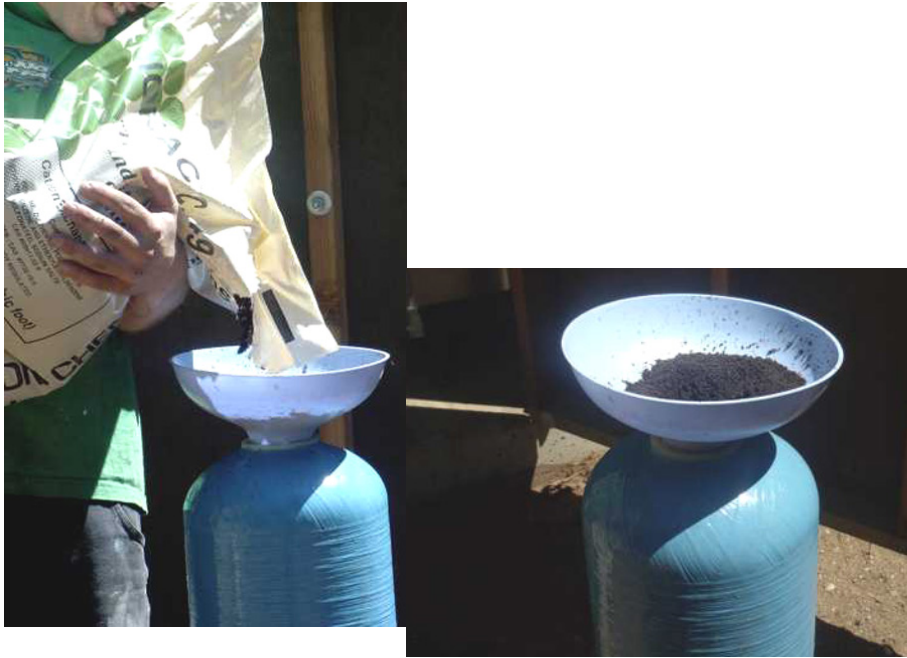
Adding resin to the tank.
