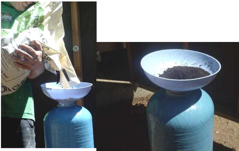
Adding resin to the tank.
