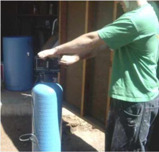
Screwing valve onto tank.
