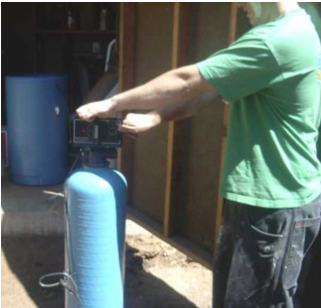
Screwing valve onto tank.
