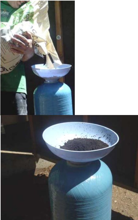
Adding media to the tank.
